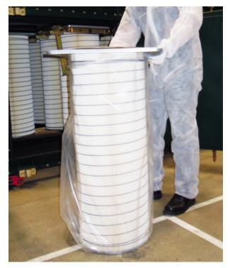
Figure 230.2.5 - Pull out the cartridge
