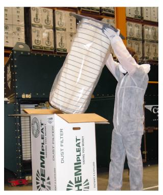
Figure 230.2.6 - Place the used cartridge in the box that came with the replacement cartridge
