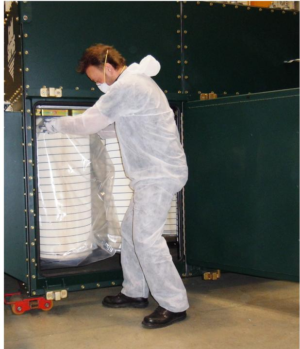
Figure 230.2.3 - Pull the bag up over the cartridge
