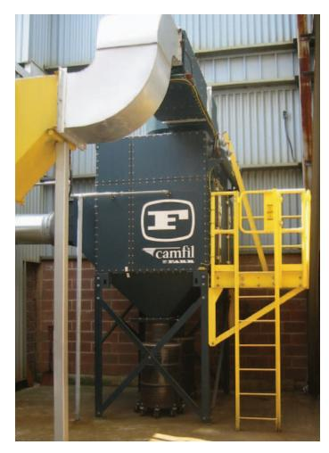
▲ A new GS12SQ was installed to replace an old, fire-prone unit.
