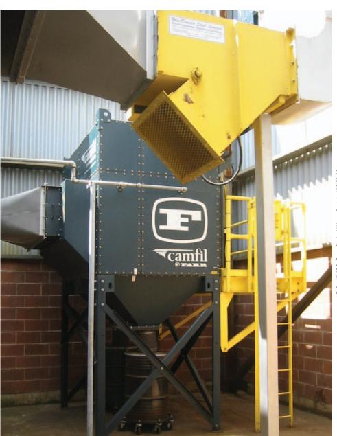
▲ The GS12SQ, fire-retardant filters and backdraft damper (installed in the ducting above the unit) have made the Héroux-Devtek completely fire and smoke free.
