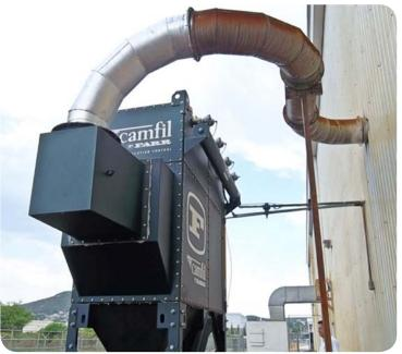
▲ Included is an abrasion-resistant inlet that works well for shot blasting.
