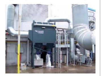
Entek chose Camfil Farr Gold Series<sup>®</sup> dust collectors ahead of strong competition because of the high efficiency and low pressure drop of the HemiPleat<sup>®</sup> filter cartridges. This together with the extremely quick filter change of the Gold Series and the low cost of replacement filters, compared to the DCE Sintamatic units, made the Gold Series the obvious choice, with payback being as little as one year.
