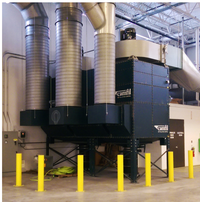
With the Gold Series dust collector, the facility stays clean and clear of dust and fumes.
