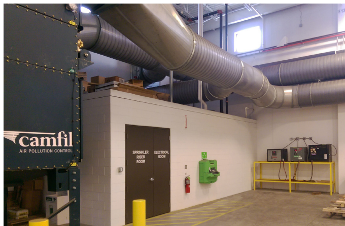
Vented ductwork runs through the entire factory to ensure the circulation of clean air.
