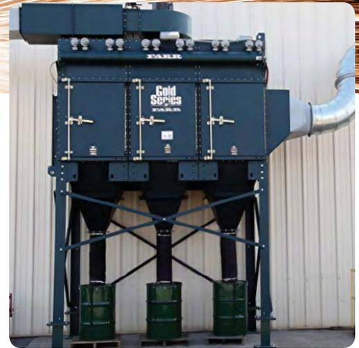
GS24 on laser cutting for carbon steel
