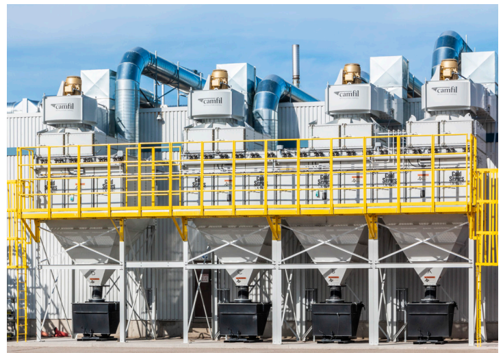
GSX144 (4-GSX36) on Robotic Weld Fume at Dyna-Mig
