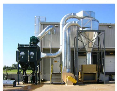
late without plugging. A dampered, top-mount fan would regulate the negative pressure to equalize the positive pressure created by the remote-mount fan pushing through the cyclone. A rupture-type explosion vent was supplied as a precaution for this potentially hazardous application.
