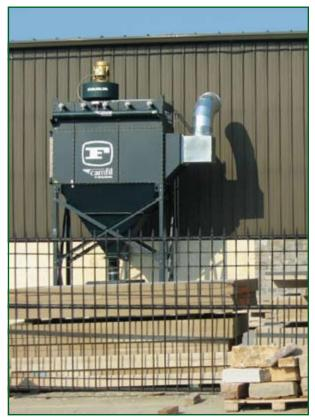
The new GS10 delivers the same amount of air as the larger, older Tenkay with less filters and lower pressure drop.
