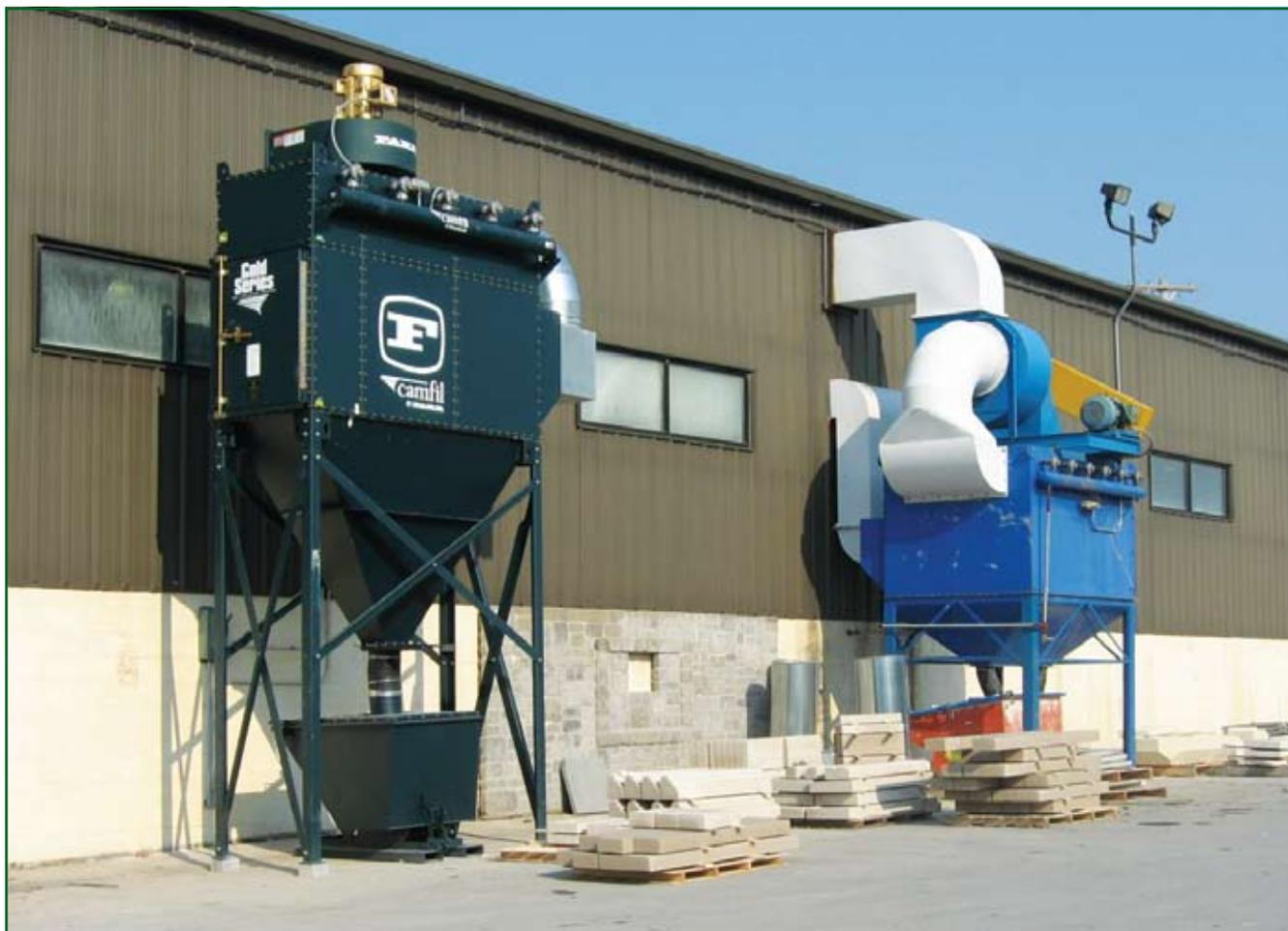
*Gold Series model GS10 relieves the particle load once captured solely by the older, undersized Farr Tenkay collector.*
