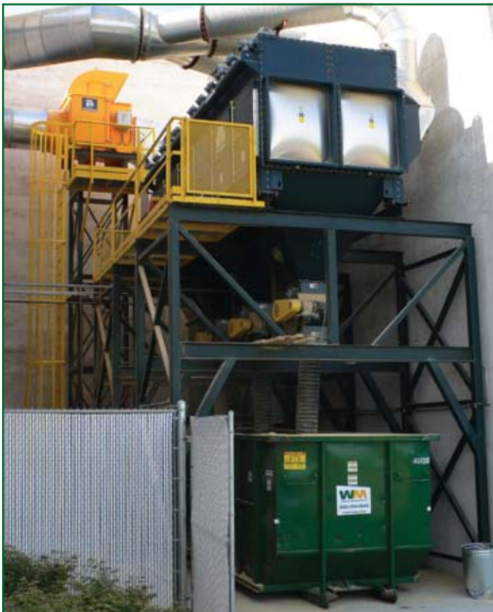
A wall was built on the side of the Gold Series collector that faced a residential area to reduce the noise level.
