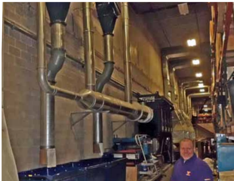
Facility Supervisor, Marlyn Mosher at Precision Press Inc. stands in foreground of the Gold Series® GS16L dust collection system.
