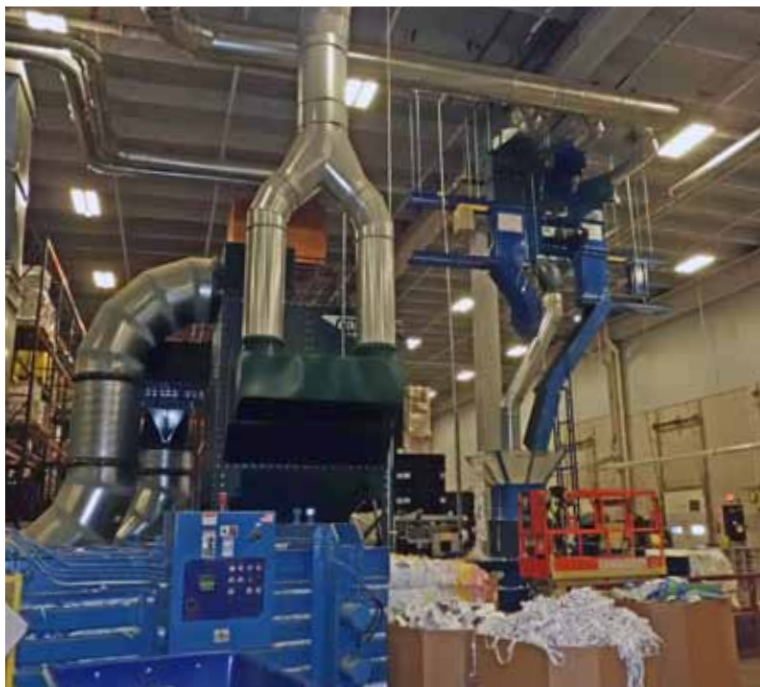
The Gold Series® GS24 industrial dust collector located near the baler and APS units.
