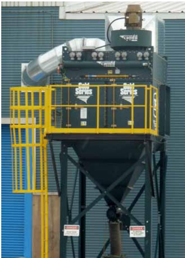
Gold Series GS20 dust collector installed at Masterloy Products Company on metal dust application.
