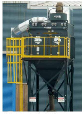
Gold Series GS20 dust collector installed at Masterloy Products Company on metal dust application.
