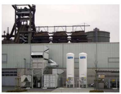
The GS40 is installed outside the factory providing more space, less noise and a cleaner working environment.
