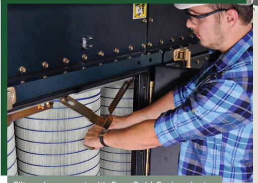
Filter change-out with Farr Gold Series dust collectors is simple and easy.
