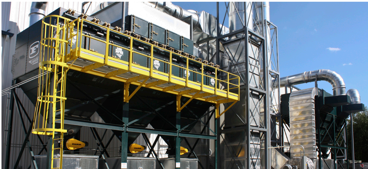
▲ The Farr Gold Series GS108 (left) is used for sand collection. The GS96 (right) is used for metal fume collection.
