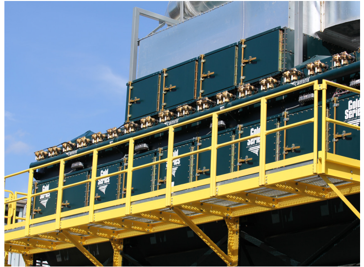
▲ The GS108 and GS72 have HEPA filters installed to return air into the building.
