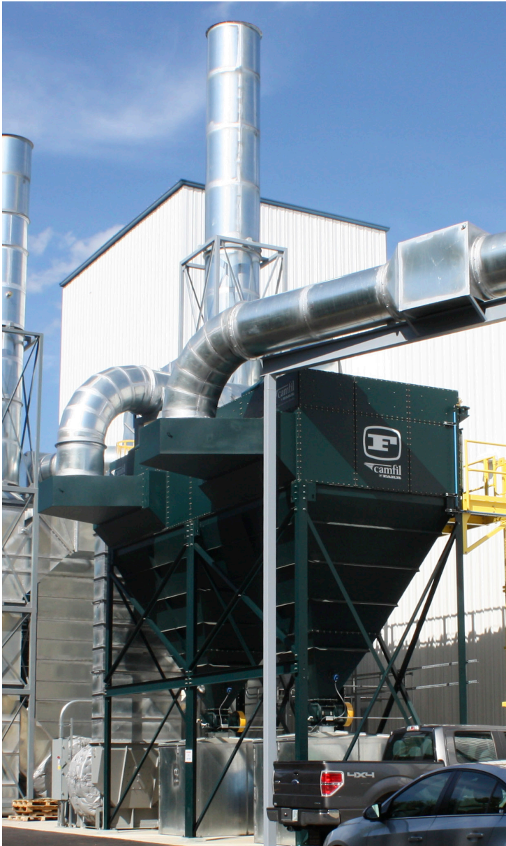
▲ A Farr Gold Series GS96 is used for metal fume collection.
