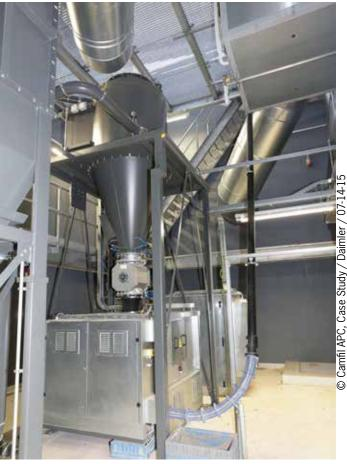
Central high-pressure vacuum filters with integrated compactor press and briquette conveyor
