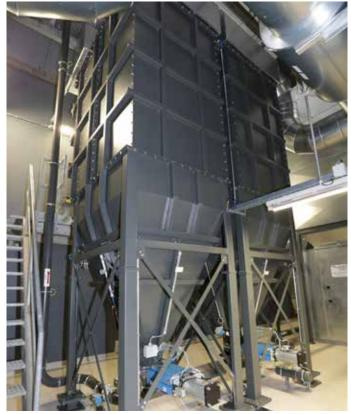
Four modular MF-ULTRA 194.3.1 units, each with 12.500m<sup>3</sup>/h volume for extraction of the milling machines with pneumatic dust and chips removal system
