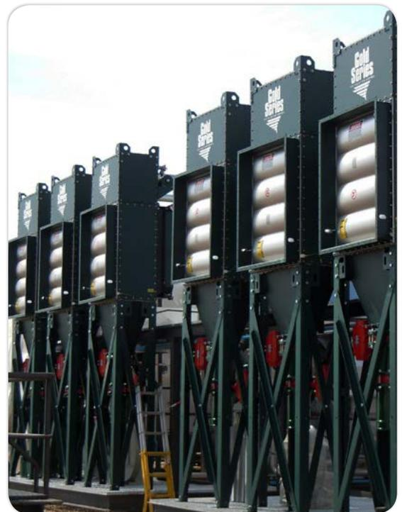
Six GSC2 Farr Gold Series Camtain units installed in September 2012 to extract dust from tablet machines at the multinational pharmaceutical company in Spain.
