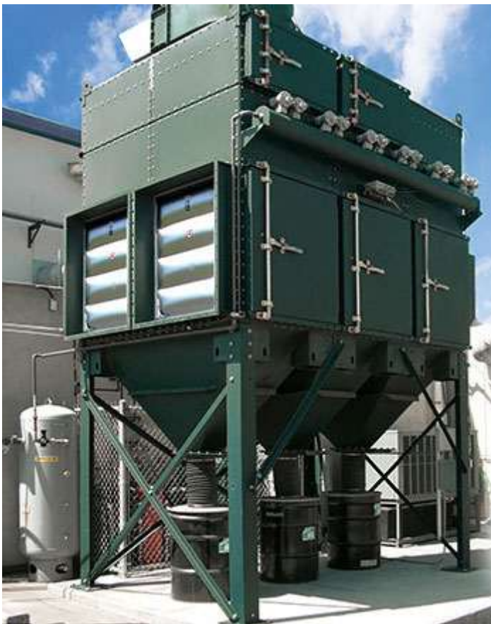
Industrial dust collector with explosion vents. Photo: Camfil APC
