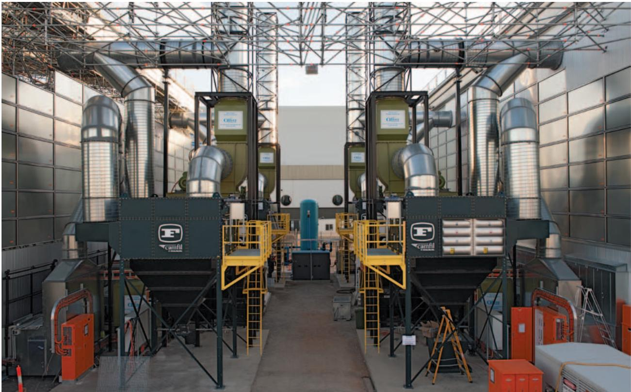
Four Farr Gold Series dust collectors with explosion vents are located between the two temporary buildings with no interference with surrounding equipment.
