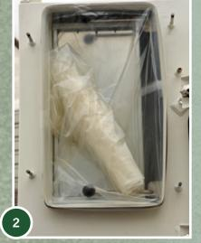
BIBO Safe-Change HEPA Filter: BIBO filter change. Ensures safe-change with the finest, most harmful dust particles.
